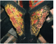
Fig.6 the combo brackets of the 'Trieu To Mieu' Ancestor Hall
